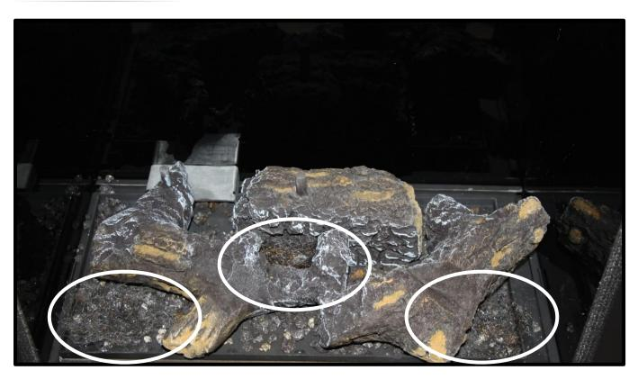
Tease out half of the Emberglow to make a very loose network of fibres and place in the spaces between the shapes and above the burner ports as highlighted.
