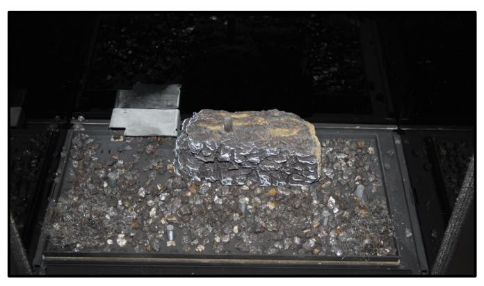
Spread a thin layer of vermiculite over the burner surface, taking great care not to block the pilot area.
