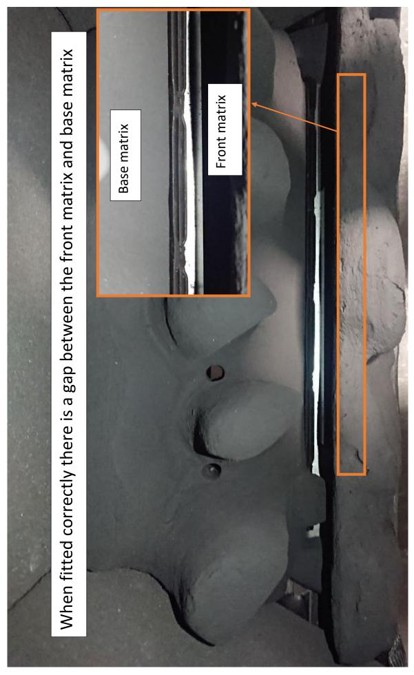
When the base matrix is fitted incorrectly the burner is covered and this will cause the components underneath to overheat causing failure of parts, also when fitted like this it exposes the metal work of the burner carrier at the back of the fire.
