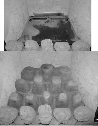
Place the first row of 3 x A and 3 x B overlay loose coals as shown between the front coals and base matrix. Make sure that they are stable and DO NOT let them fall down in the gaps between the peaks on the matrix.
