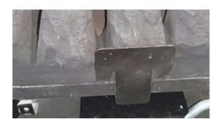
• Place the front row of six coals, as shown. Ensure these coals are supported by the front Matrix and the rear matrix and will not wobble or fall through on to the burner. This row is important to support the next rows properly. If necessary turn upside down and rotate to find stable positions. The positions shown in the photograph should be suitable.
