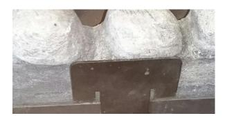
Place the first row of five large pebbles as shown. So that they sit on the Front Matrix in the indents provided. Check that they are stable against the rear matrix by putting slight pressure on them with your fingers. Reposition any that are unstable. Mix the two grey and beige colours to give a pleasing layout.
