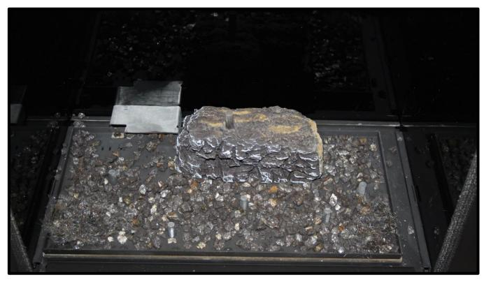
Spread a thin layer of vermiculite over the burner plaque taking great care around the pilot area.
