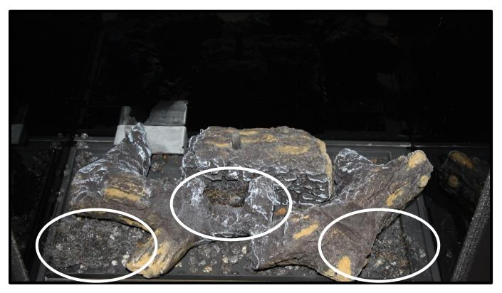
Tease out half of the Emberglow to make a very loose network of fibres and place in the spaces between the shapes and above the burner ports as highlighted.
