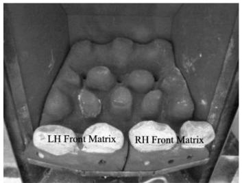
Lay one row of pebbles at the front of the fire as shown. A second row (number positioned against the rear of fire) is placed between the base matrix and the rear of the fire as shown.
