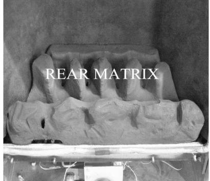
When positioning the rear matrix be careful not to cover the burner ports
