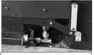
Cut a cross slit in the rubber grommet and feed the appliance onto the 8mm-gas supply pipe. Position the restrictor elbow supplied and mark supply pipe at its cut off length. Remove appliance, cut pipe to correct length, refit appliance and make gas connection with restrictor elbow use 15mm A/F spanner taking care not to apply any force to the gas control spindle as above. Ensure the restrictor valve is opened and its cap replaced tightly.
