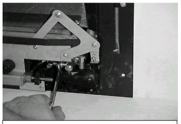
Cut a cross slit in the rubber grommet and feed the appliance onto the 8mm-gas supply pipe. Position the restrictor elbow supplied and mark supply pipe at its cut off length. Remove appliance, cut pipe to correct length, refit appliance and make gas connection with restrictor elbow use 15mm A/F spanner taking care not to apply any force to the gas control spindle as above. Ensure the restrictor valve is opened and its cap replaced tightly.
