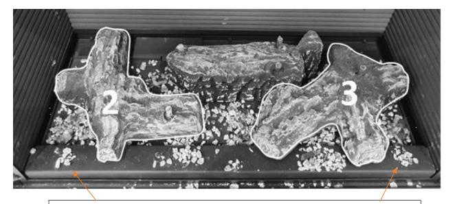
Place some of the vermiculite here along the front edge cover between the logs
