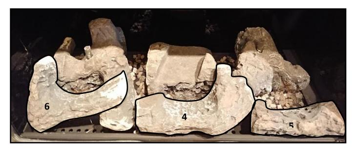
Fit the front three logs as shown.
