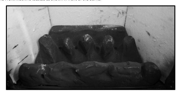
• The Rear Matrix is located so that it fits behind the burner (ensure it is not placed over the burner)
