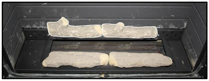
• Place a further two log shapes upon the shelf above the inlet baffle as shown.
