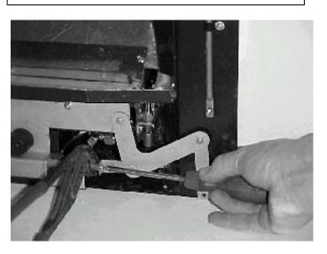
Check for gas soundness. Reconnect the bell crank mechanism as above ensuring that the gas control spindle is gripped only over the protective copper sleeve and no other part of the spindle as, ensure NO side strain is applied to the spindle.
