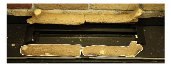
• Place a further 2 off log shapes along the front edge of the burner cover as shown.
