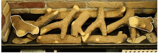
• Place the last two large shapes LH and RH as shown.
