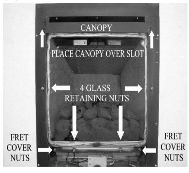
Ensure all the residues of the cleaner are removed with a damp cloth and the glass panel is completely dry before fitting to the appliance.
