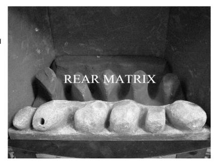
When positioning the rear matrix be careful not to cover the burner ports
