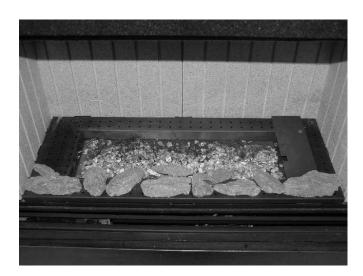
Place air tray within burner shelf assembly and cover the burner plate with a thin layer of vermiculite. (LPG ONLY)
