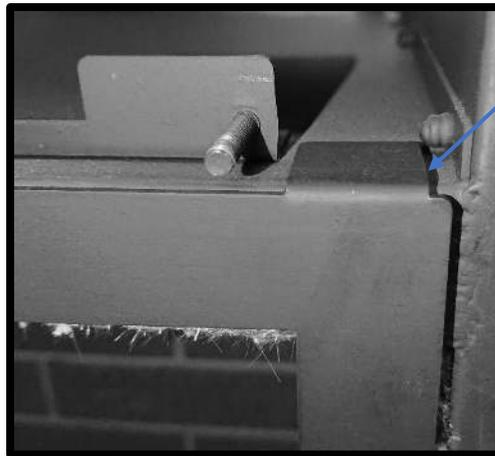
Make sure that the gap here is the same on both sides of the frame
