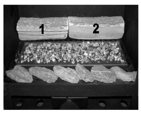
Place a single layer of Bark Chips in front of the Burner Bar making sure not to cover or obstruct the Pilot assembly or rest too far onto the Burner Bar.  Place the first Log Shape (3) as far to the right and back as possible, resting on the rear shape and resting on top of the Bark Chips as shown in the picture.
