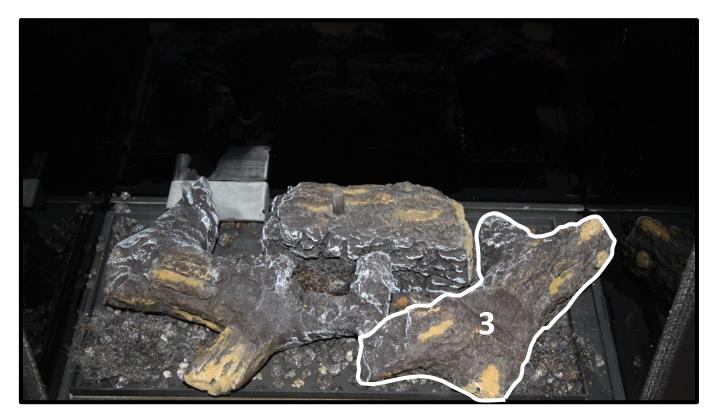
Place the final base piece on its location pins as shown.
