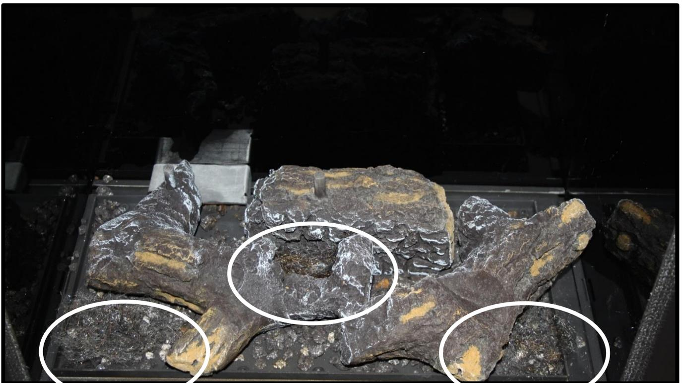
Tease out half or the Emberglow to make a very loose network of fibres and place in the spaces between the shapes and above the burner ports as highlighted.
