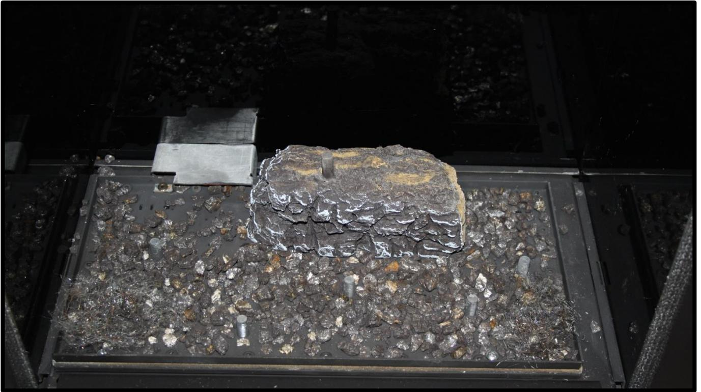
Spread a thin layer of vermiculite over the burner plaque taking great care around the pilot area.
