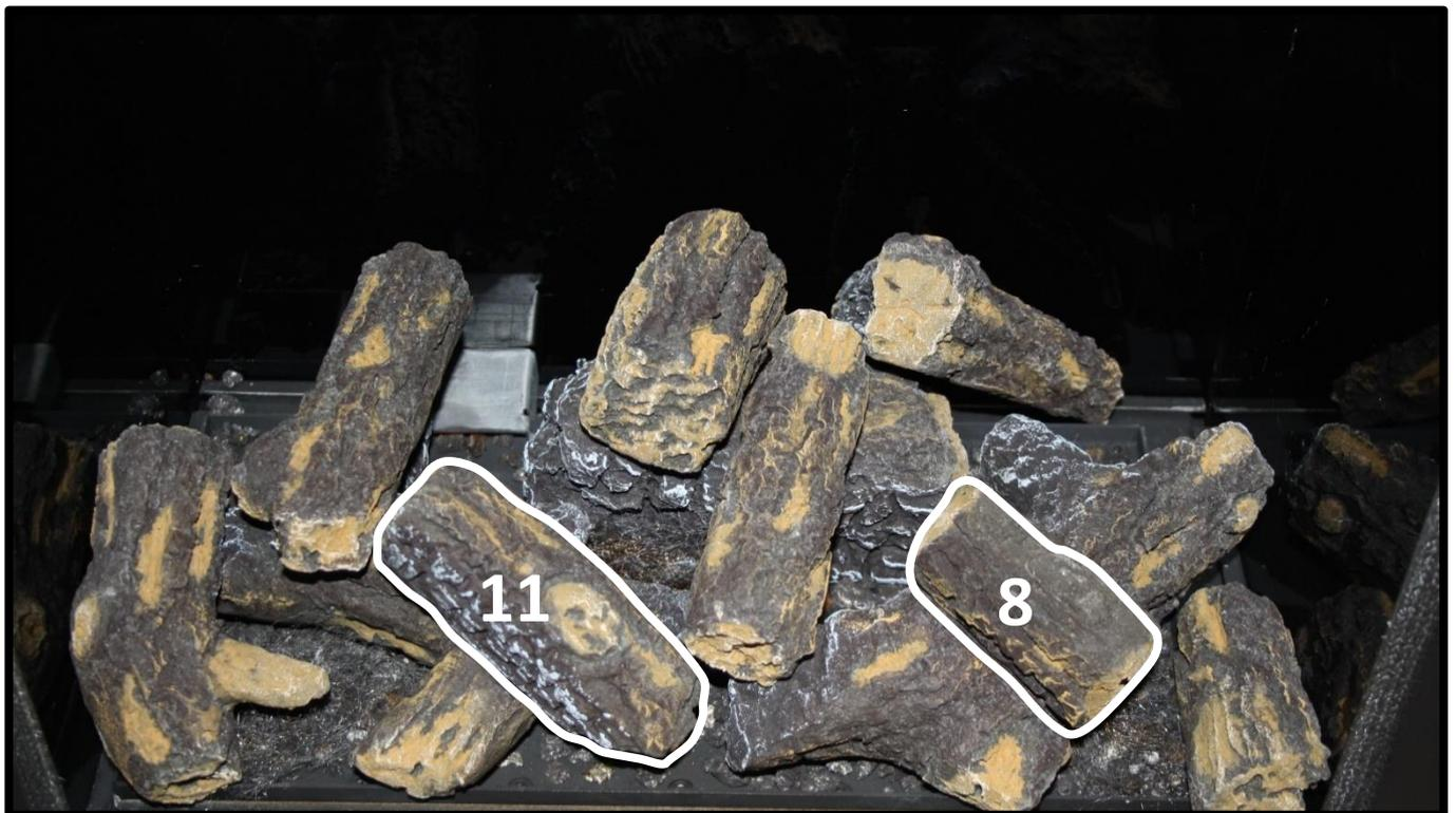
Place the final two log shapes as shown to complete the log layout.
