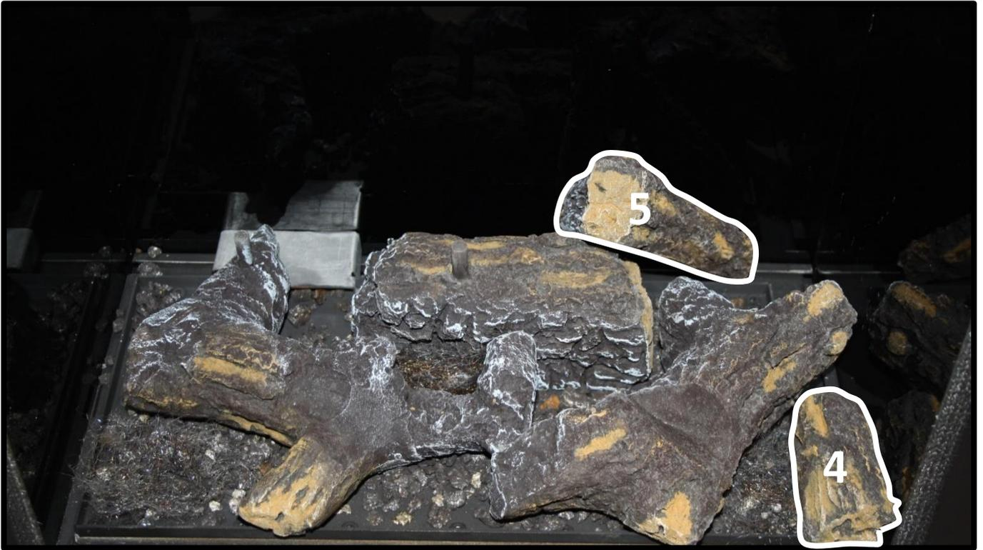
Place a further 2 log shapes as highlighted above. Log No5 is a Y shaped log.
