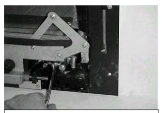
Cut a cross slit in the rubber grommet and feed the appliance onto the 8mm-gas supply pipe. Position the restrictor elbow supplied either as shown or on top of the valve to the left of the inlet elbow using the cutout provided.
