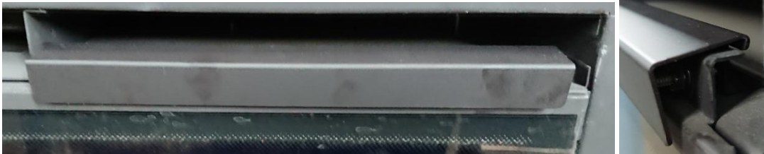
Fixing cover slides over the top of the fixing bracket and hooks over the back of the bracket
