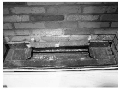
Place a further 2 off log shapes along the front edge of the burner cover as shown.
