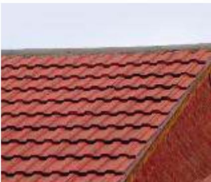
No chimney or flue
